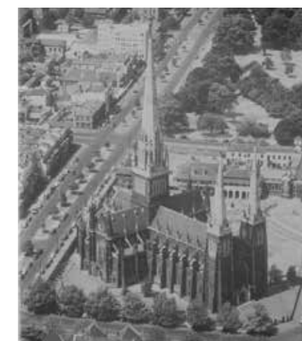
St Patrick's cathedral showing Gisborne Street and Albert Street tree plantings taken between 1930 and 1939. Gisborne Street is thought to have been planted around 1906 and the Albert Street medians were constructed and planted in the 1930s [The Rose Series, State Library of Victoria].
