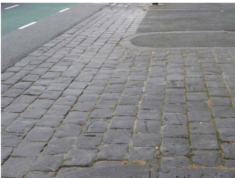
Figure 17 Bluestone crossovers, kerb and six course pitcher gutter, Queensberry Street, 2010.
