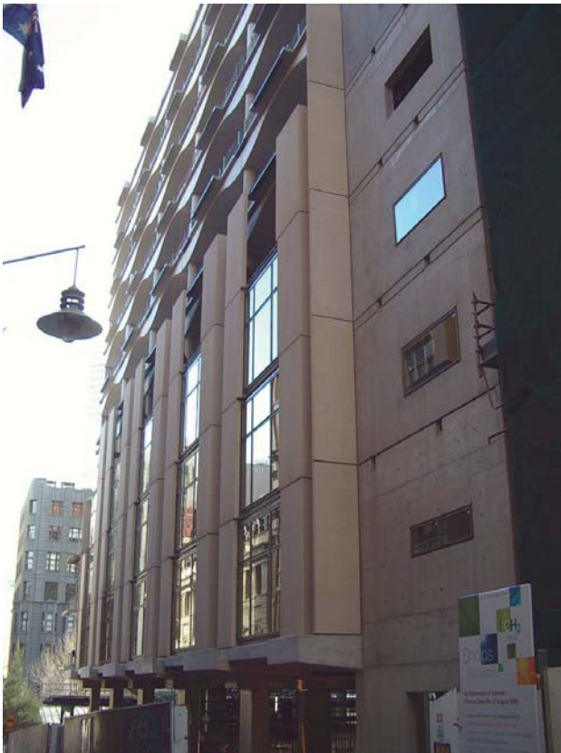
C. South façade view, August 2005.
