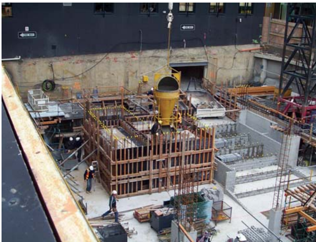
A. Car park access link to adjacent building, October 2004.
