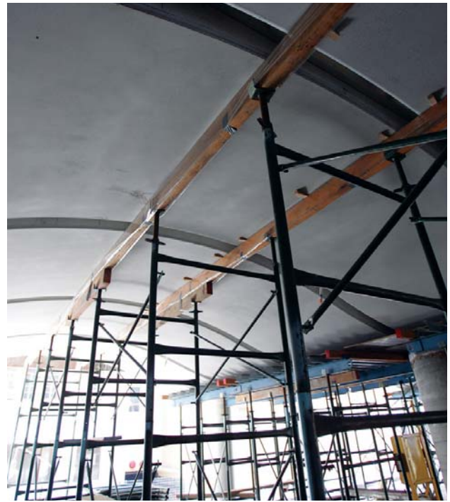
A. Apex of curve with structural support.
