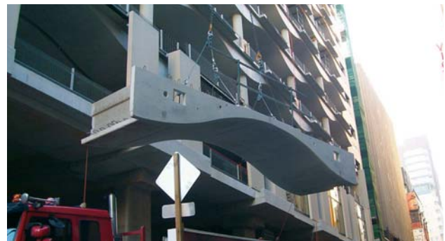
B. North end panel, note square penetration for ventilation exhaust (refer Figure 3B).
