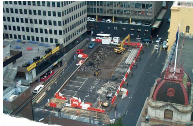
B. Site at start of construction, February 2004.
