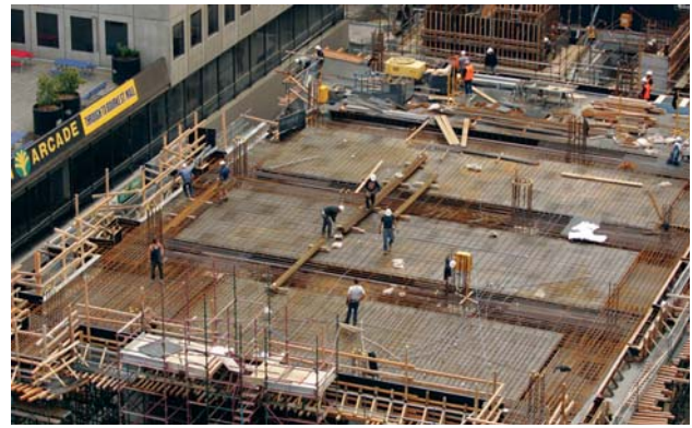
C. First floor formwork, November 2004.
