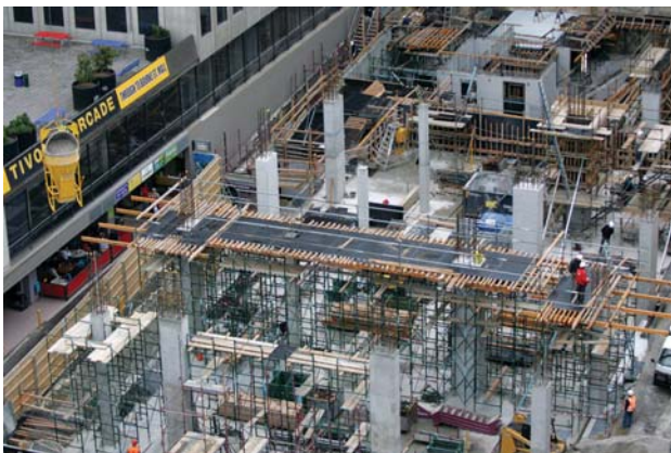
B. First floor under construction, September 2004.
