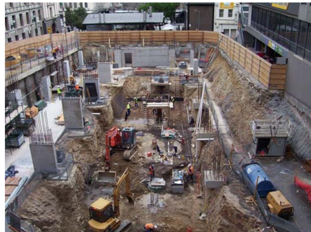
C. Site excavation, August 2004.
