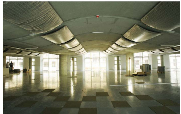
C. Positioning tile pattern on raised floor.
