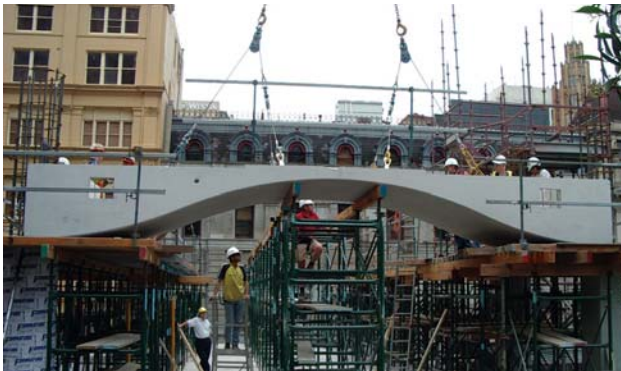
D. Ceiling panel with supports.
