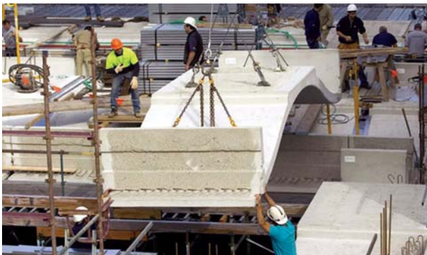
E. Placing central panel.
