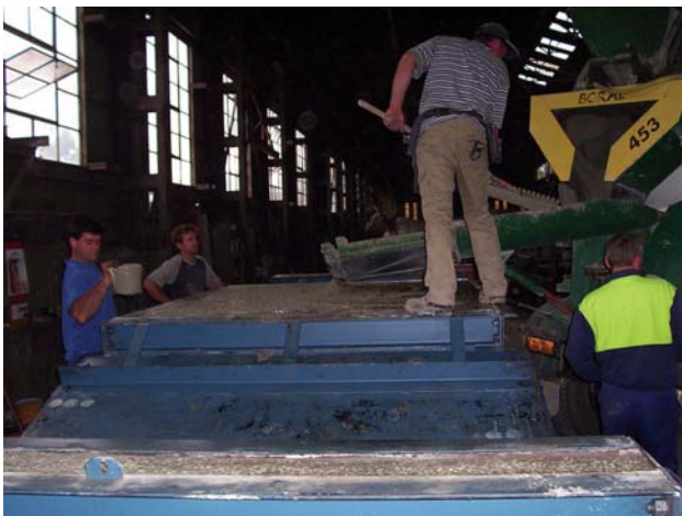
C. Pouring concrete into mould.
