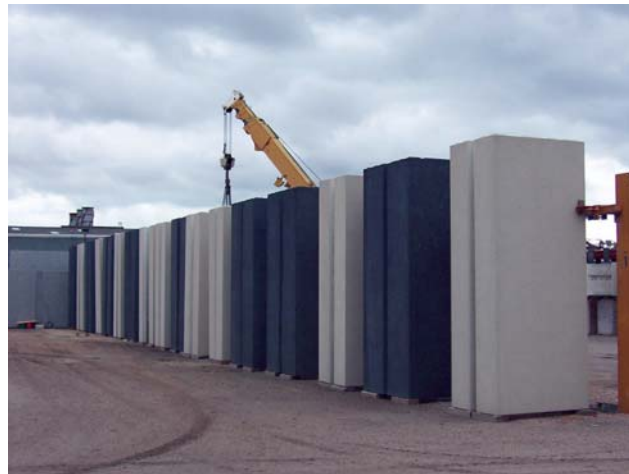
B. Panels awaiting delivery to construction site.
