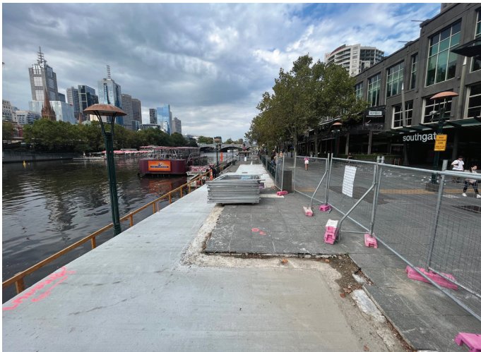
Works at the western end will recommence shortly
