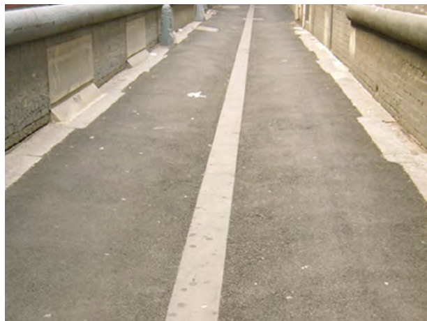
Sawn bluestone channel
