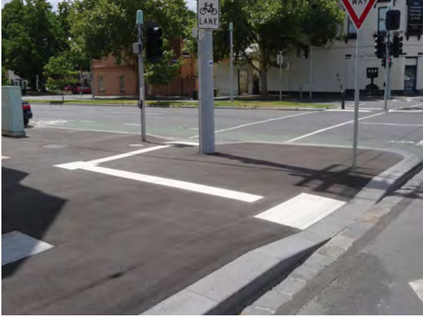
Access ramp typical corner asphalt footpath
