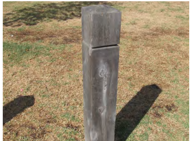
Timber bollard - fixed
