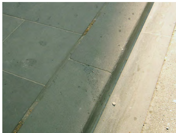
Sawn bluestone kerb and gutterstone
