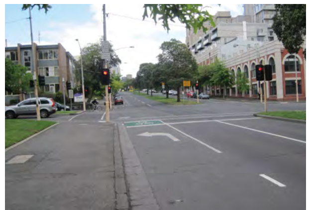
Asphalt road pavement
