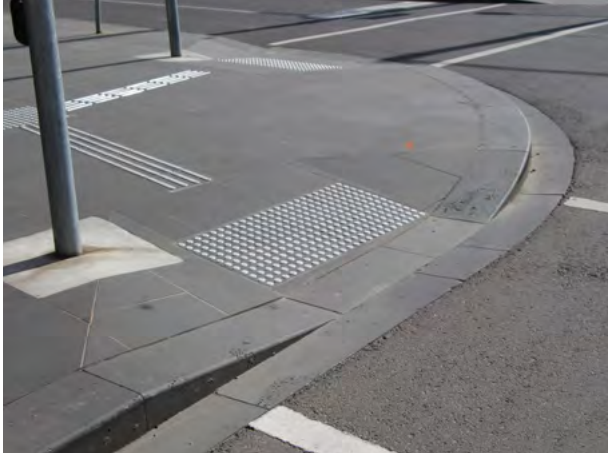
Access ramp typical corner bluestone footpath
