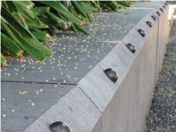
Skate deterrent bronze button ↖ Design Standard 705.04
