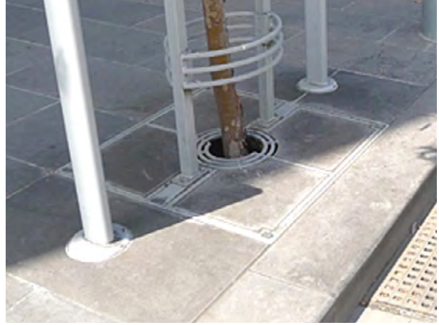
Tree pit bio-retention type in bluestone paving
