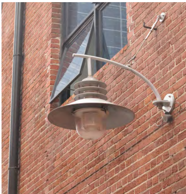
In narrow streets and laneways, wall-mounted lights should be used to keep limited footpath space clear for circulation. Light poles in these situations are also liable to damage since space for manoeuvring vehicles is tight.
