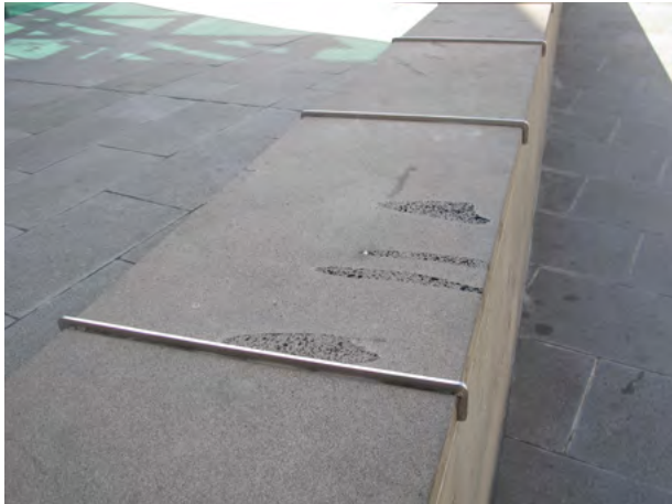
Skate deterrent long fin ↖ Design Standard 705.01
