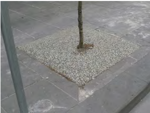
Tree pit standard size in bluestone paved area
