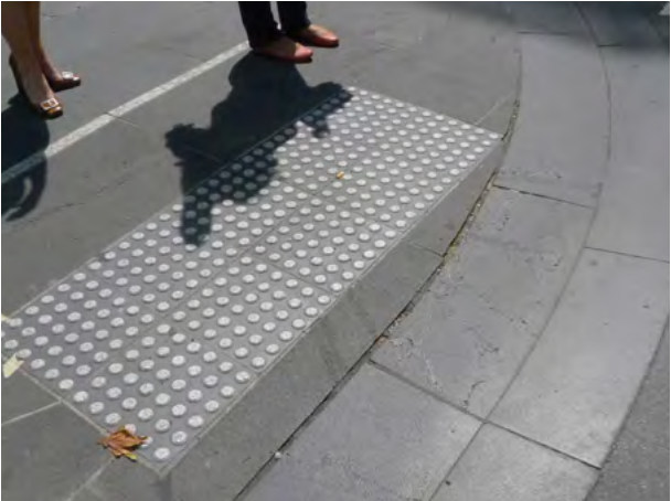
Access ramp joined narrow bluestone footpath
