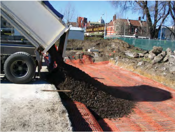
Tree pit in combination with structural soil
