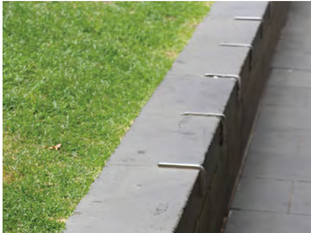
Skate deterrent short fin ↖ Design Standard 705.02
