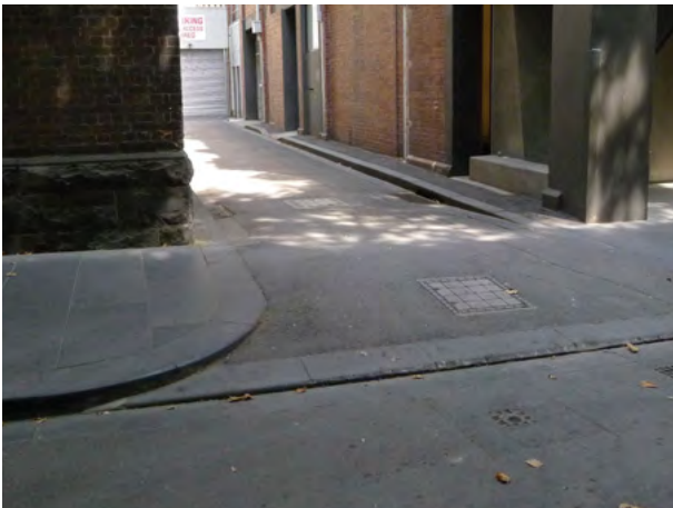
Crossing asphalt paving for laneway with side pits
