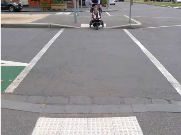
Access ramp for median/island
