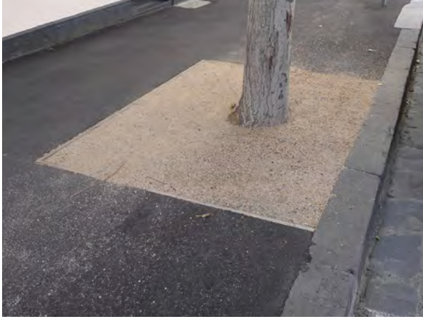
Tree pit in asphalt paved area
