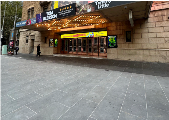
Wider footpath and new bluestone pavers in front of the Comedy Theatre
