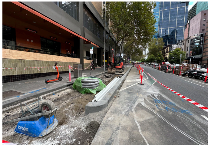
Works underway in front of Rydges Hotel
