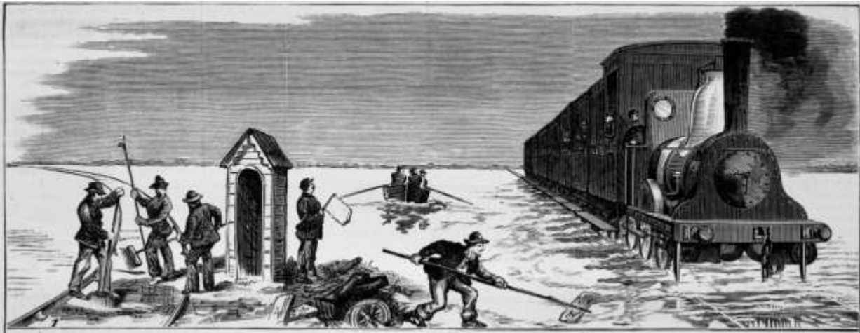
Figure 38: Floods along the Port Melbourne Line 108
