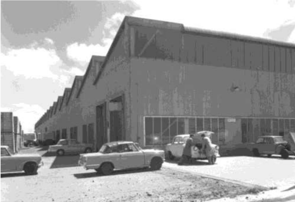
Figure 58: External view of the Standard Motor Products factory, 1962 142
