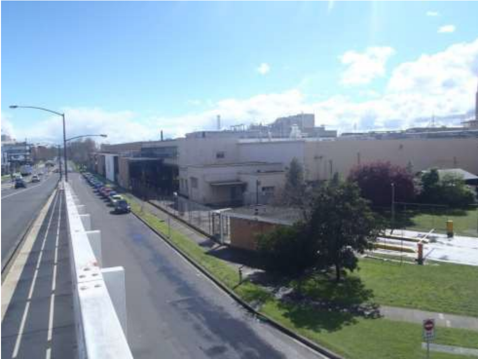
Figure 67: View of Kraft Factory from Salmon Street overpass
