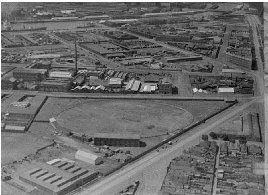
Figure 19: View to east from near Port Melbourne Football Ground showing Kitchen & Sons and warehousing/timber yards beyond.
