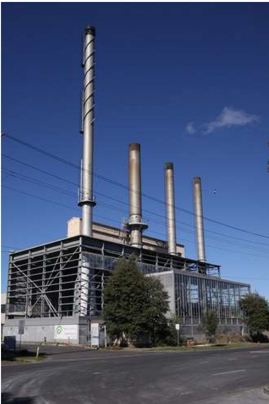
Figure 54: Demolished Holden Boiler House (Photo Wongm)
