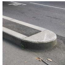
Concrete separator island
