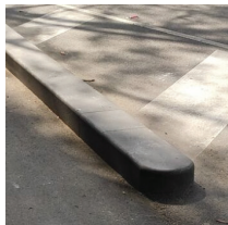
Concrete separator kerb
