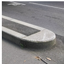
Concrete separator island
