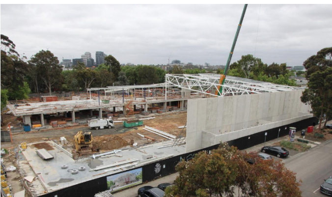
Aerial view of the construction site
