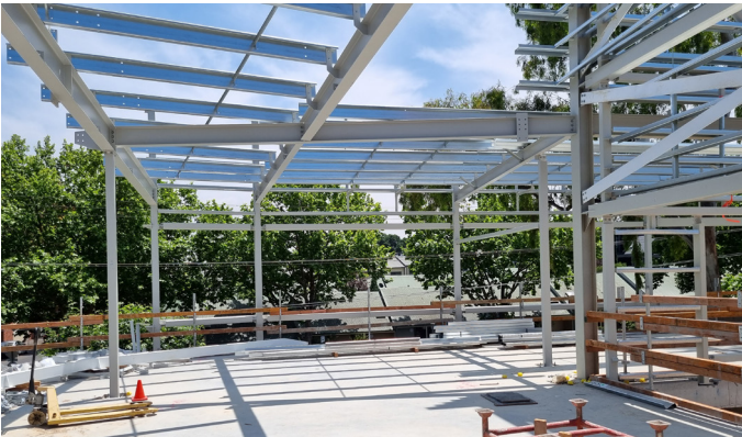
Metal framing for the stadium
