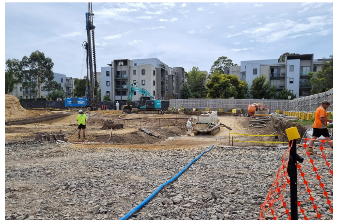
Soil removal works continue on site
