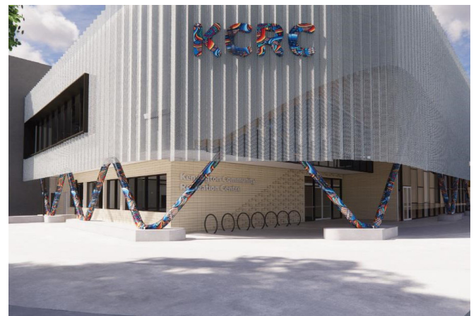
Entrance to new centre
