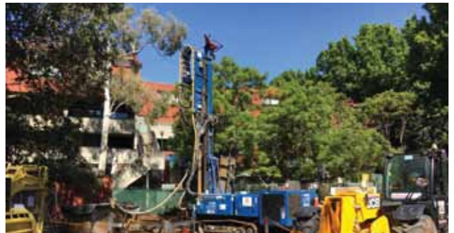
Above and below - specialised drilling rig to install the 100m deep geothermal bores
