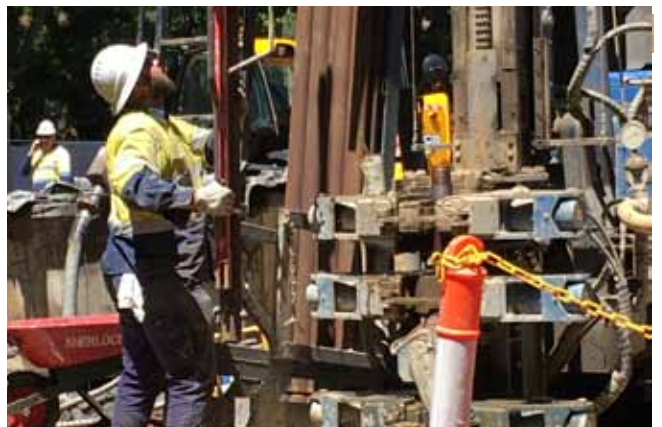
Above and below - specialised drilling rig to install the 100m deep geothermal bores
