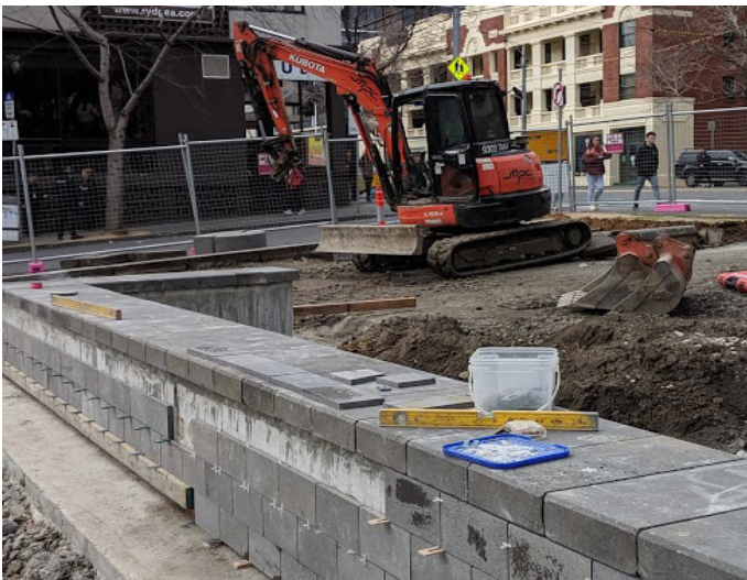
New retaining wall construction at Lincoln Square South
