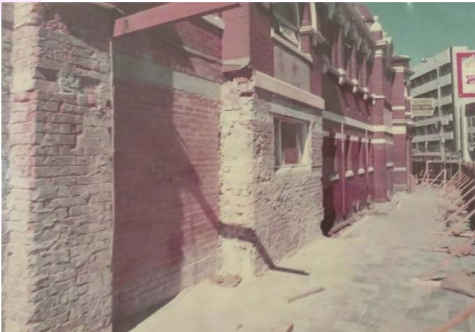
FIGURE 53 THE BOILER HOUSE WAS DEMOLISHED DURING THE 1981-3 WORKS
