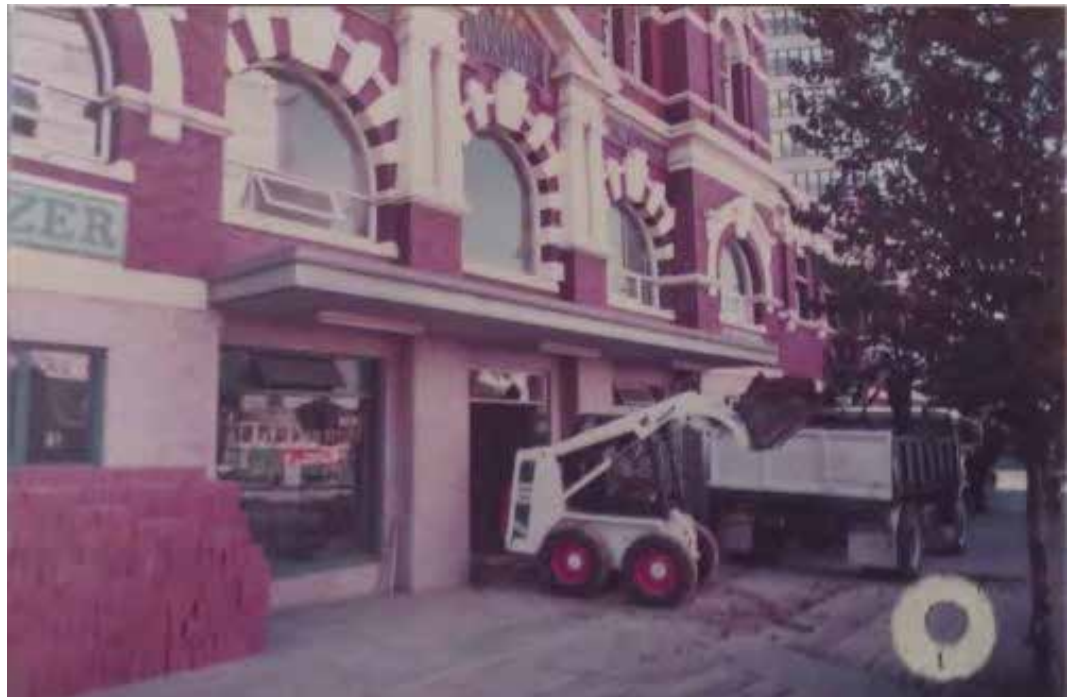
Figure 39 A photograph taken during works in the early 1980s to remove the 1960s façade
