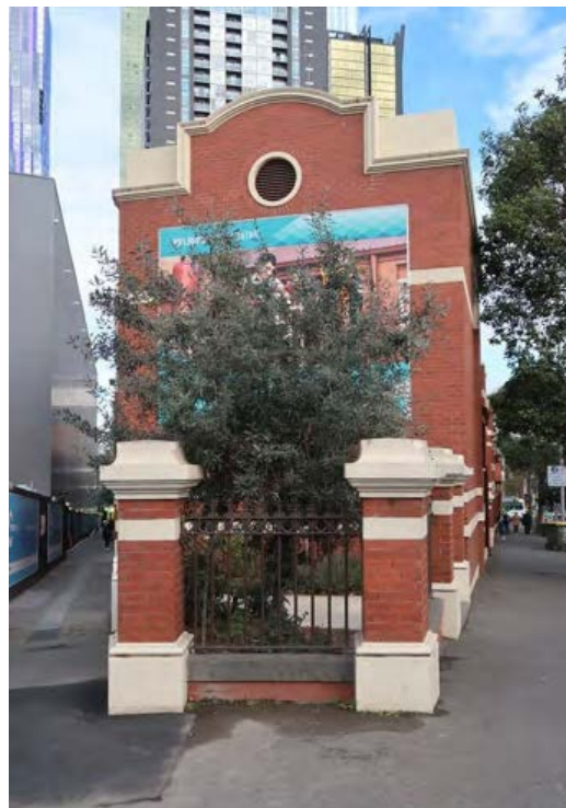
Figure 65 (a) Franklin Street façade; original windows to the pool survive in the western section of the façade; (b) the junction of original and 1980s fabric
