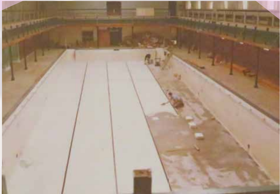
FIGURE 44 THE MAIN POOL IS RESURFACED, EARLY 1980S
