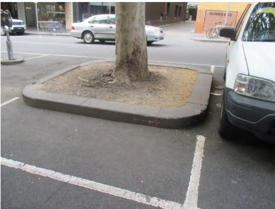
Figure 33: Bluestone kerb tree island
