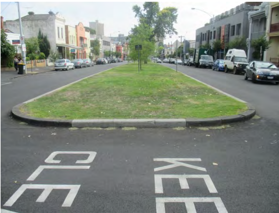
Figure 35: Median constructed in exposed aggregate precast concrete kerb retaining old bluestone kerb radials
