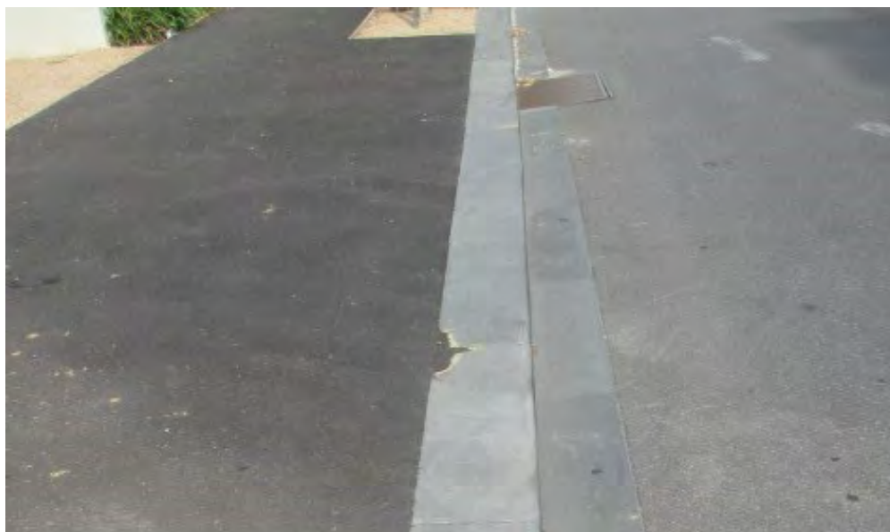
Figure 30: New sawn bluestone kerb and channel installed adjacent to asphalt footpath
