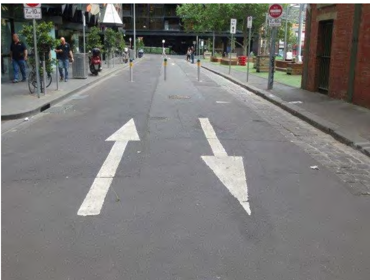
Figure 20: Stewart Street – footpath widening required removal of the wide pitcher channel
