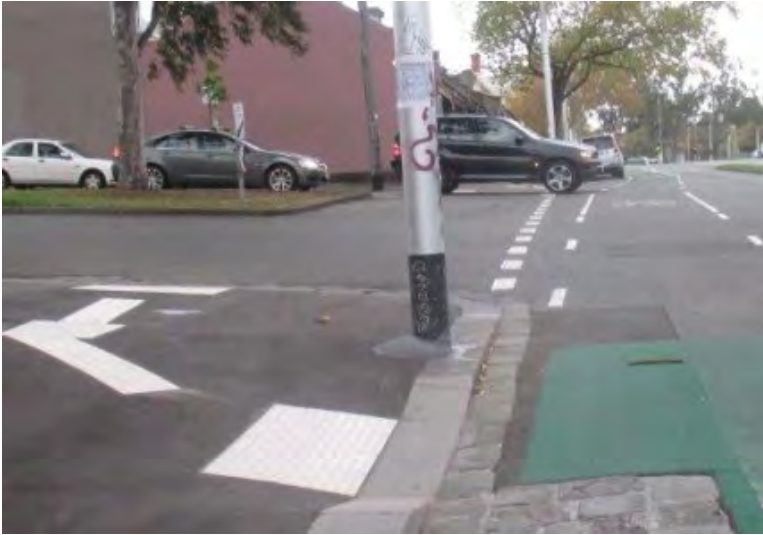
Figure 18: Abbotsford Street North Melbourne – Four row wide pitcher channel reduced to a single row to accommodate an access ramp and bicycle lane (Heritage Overlay Area)
