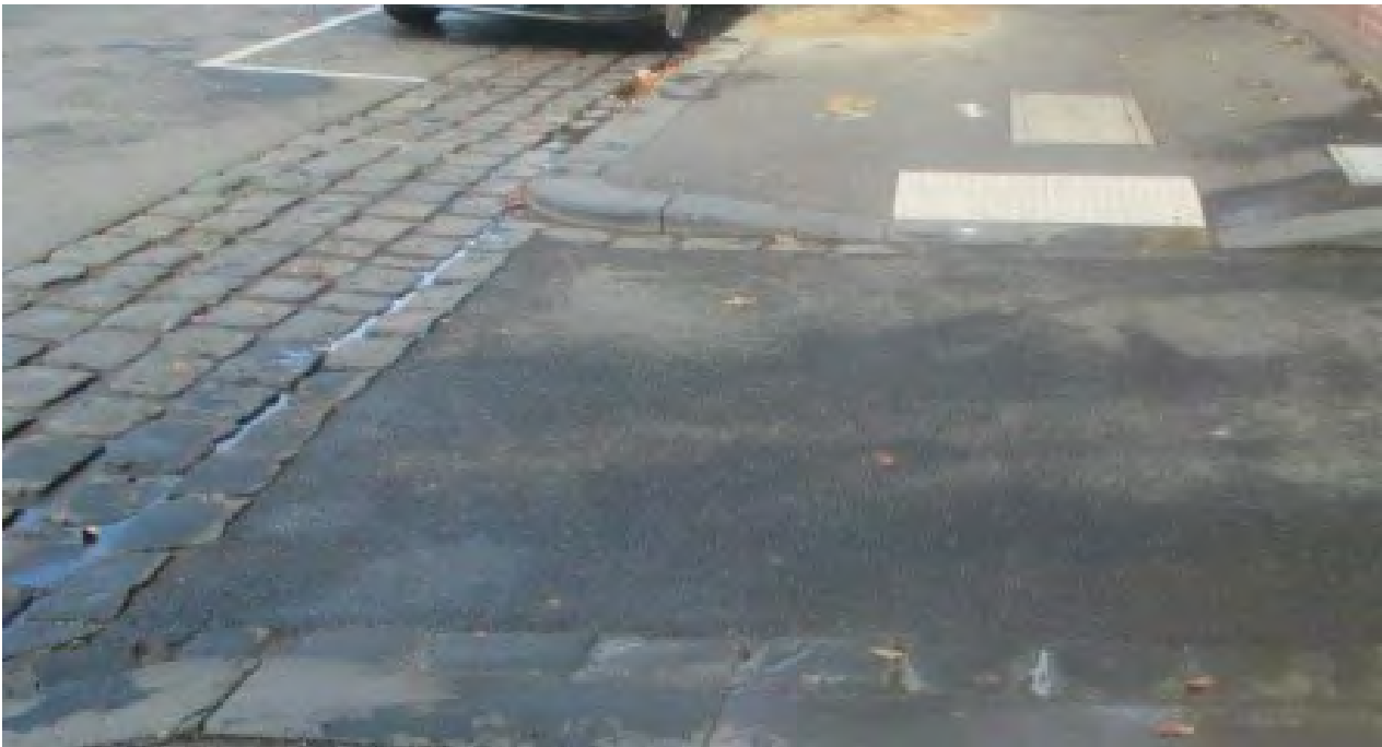
Figure 14: Bluestone Pitcher Laneway in Heritage Overlay area – Crossing constructed in asphalt due to Disability Discrimination Act requirements (c.2000)
