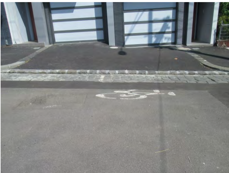
Figure 37: Crossing reconstructed in asphalt
