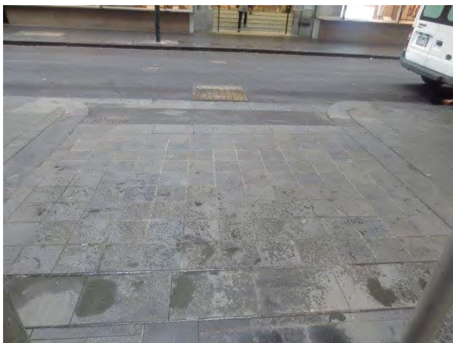
Figure 23: Driver Lane – crossing reconstructed in sawn bluestone paving blocks – built 2014
