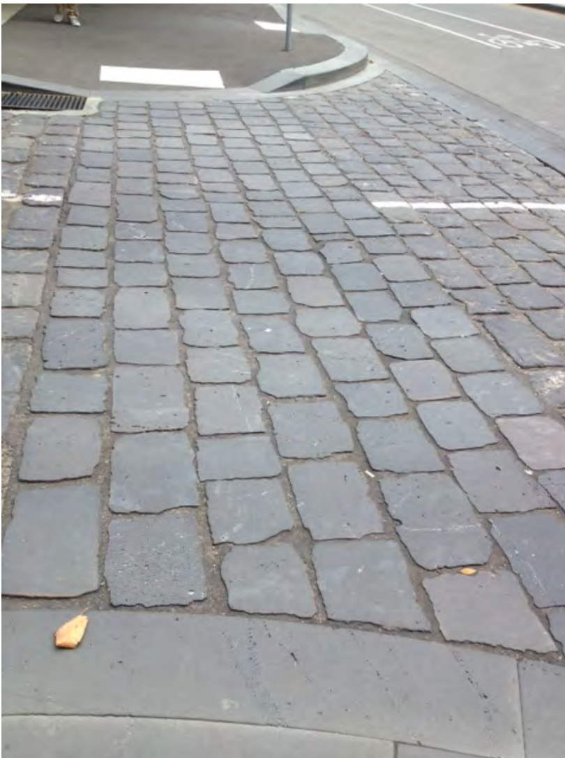
Figure 10: Sawn bluestone pichers used at the intersection of Merchant and Bourke streets, Docklands, to make the crossing wheelchair accessible. Built in 2013.
