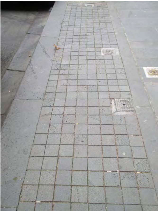
Figure 25: Use of permeable sawn bluestone sets at the edge of a footpath
