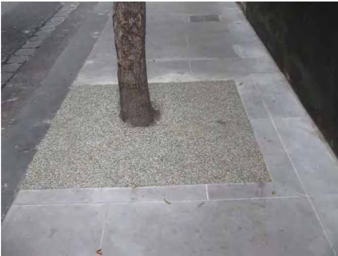
Figure 24: Use of permeable 'pebble' style paving in a tree plot
