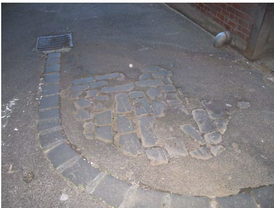
Figure 2: Evidence of the original bluestone pitcher laneway beneath the deteriorating asphalt surface
