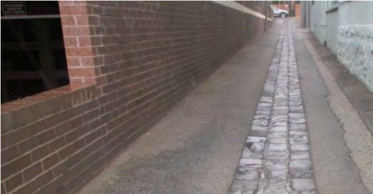
Figure 15: CL 1448 off Domain Road – pitcher laneway reconstructed in asphalt in response to a request by a resident to provide Disability Discrimination Act access (Heritage Overlay area). Built circa 2000.
