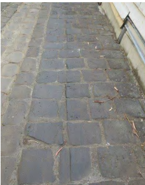
Figure 9: CL0182 (Heritage Overlay Area) – Reconstructed in 2007 (showing an approximately 10m length of 'cart tracks' reinstated as a sample of tracks that previously existed)
