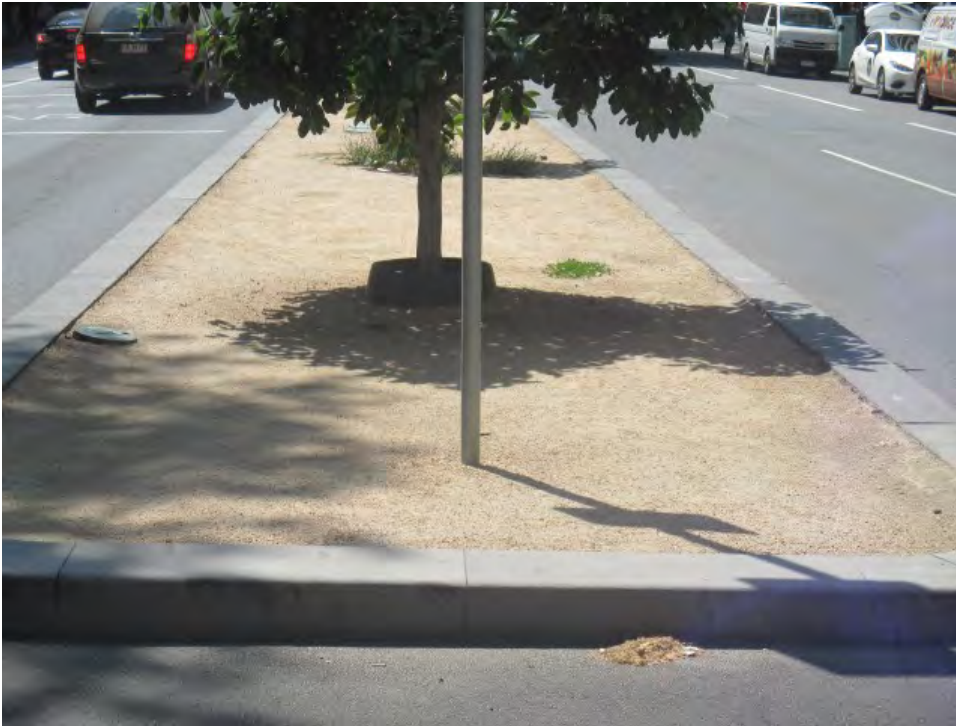
Figure 32: Median constructed in sawn bluestone with granitic gravel infill
