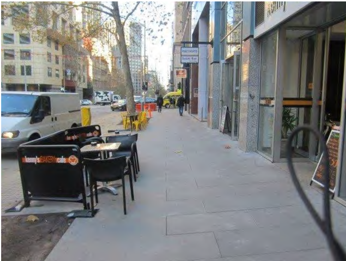
Figure 21: New sawn bluestone paving
