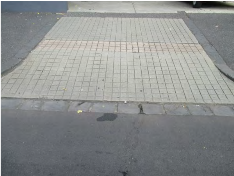
Figure 36: Crossing reconstructed in concrete
