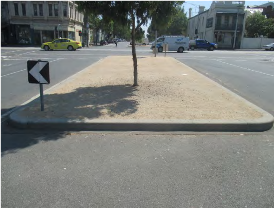
Figure 34: Median constructed in exposed aggregate precast concrete kerb
