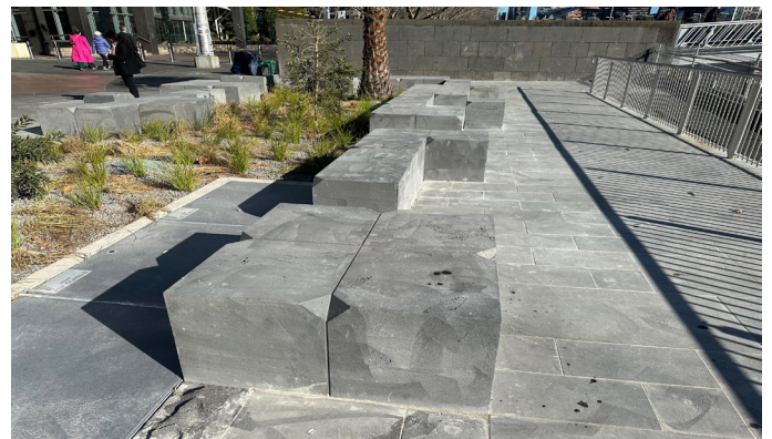
The recently completed works
