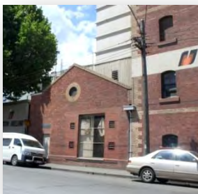
Figure 124 Northern extent of complex, gabled store contributory part of complex
