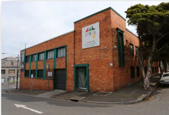
Figure 172 Corner view from south showing new central shuttered opening , 2013
