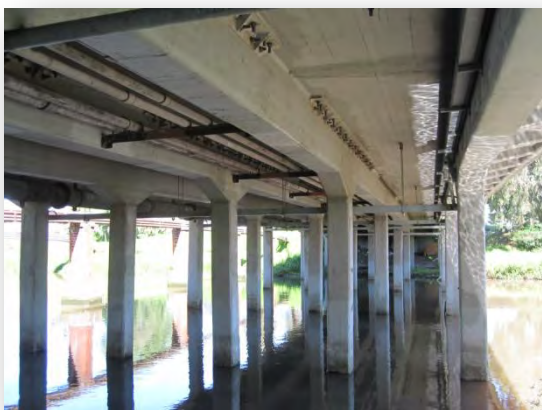
Figure 59 reinforced concrete substructure from east end
