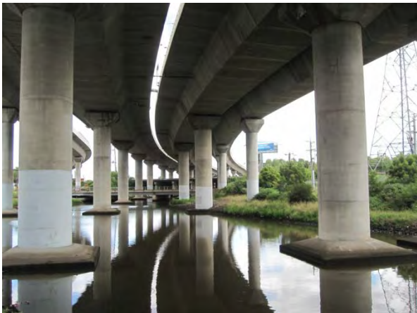
Figure 193 Under Citylink, looking north
