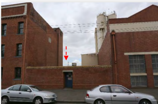
Figure 20 Wall in Munster Terrace with new opening, appears Victorian-era - rear of Building 3.
