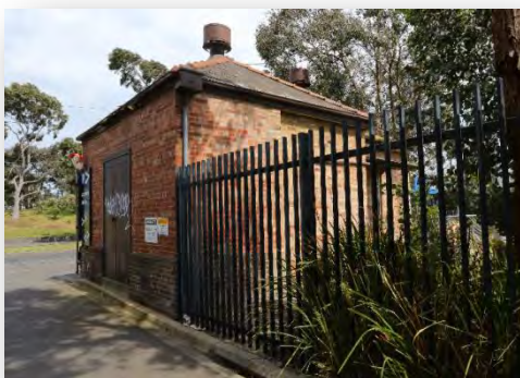
Figure 146 Rear view of altered caretaker's house.
