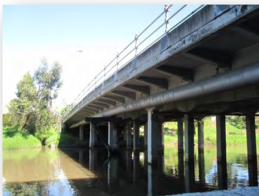
Figure 160 Bridge structure and pipe way, 2011
