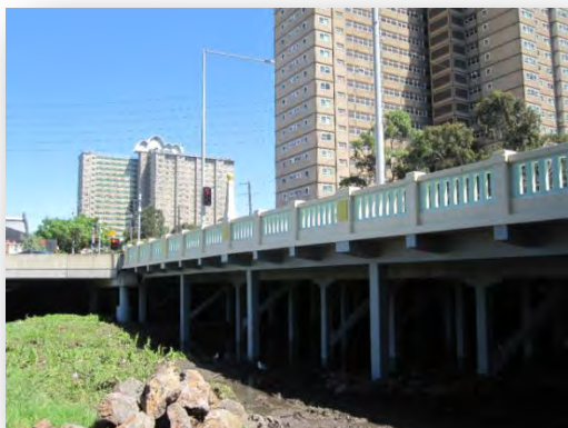
Figure 216 View from south
