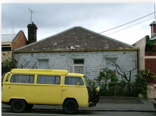
Figure 102 House in 1990s, with original slate roof.
