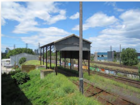
- Figure 68 Siding shed to west
