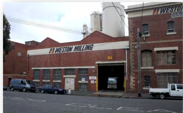
Figure 126 inter-war infill south of Brunton mill in 1-25 Munster Terrace.
