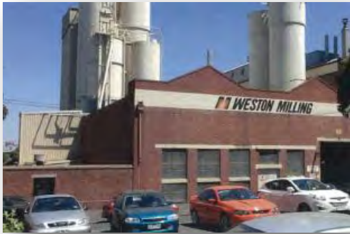
Figure 19 Munster Terrace Wall and Building 3 (Raworth)
