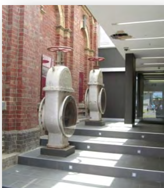
Figure 151 Regulator valves in new development adjoining valve house, 2011
