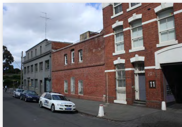
Figure 10 Anderson Street elevations, part existing heritage overlay: Smith & Sons later Brockhoff biscuit factory and rd brick TB Guest biscuit factory wings , 2011
