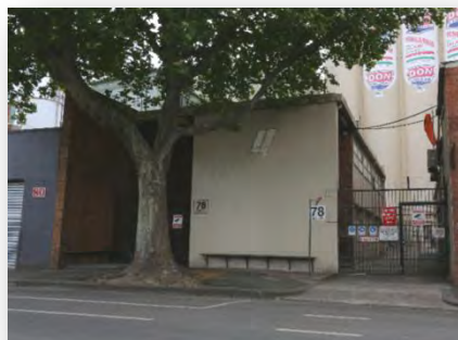
Figure 24 Offices 78 Laurens St, Building 6
