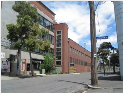
Figure 63 Mill and store seen from east, with altered mill (east wing)
