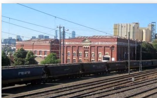
Figure 111 View of stores 2, 1 from north, 2012, train in siding
