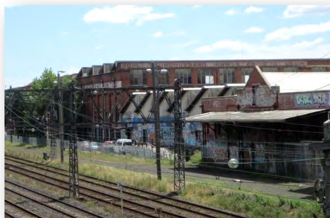
Figure 116 West elevation from south, sawtooth store 5
