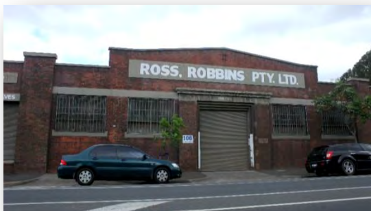
Figure 224 View from south-east (Google)
