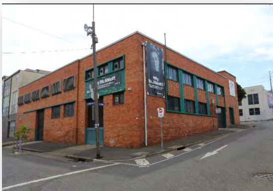
Figure 173 Corner view from south, showing Modernist fenestration patterns, undisturbed by changes
