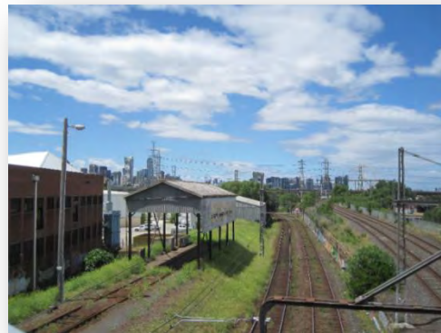
Figure 69 Siding and shed from footbridge
