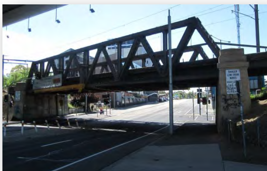
Figure 212 Bridge from west, showing trusses and rendered pylons.
