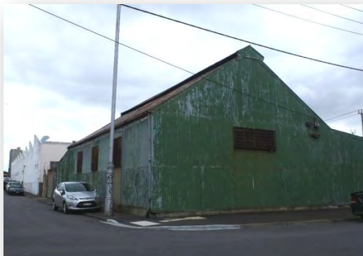
Figure 220 View from south
