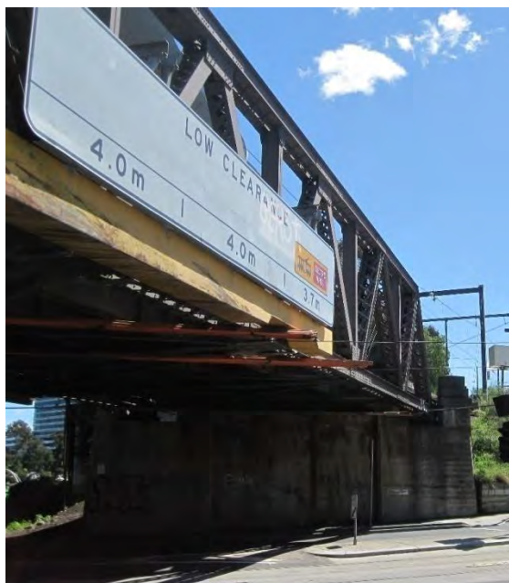
Figure 213 From north end, with added signs and safety guard
