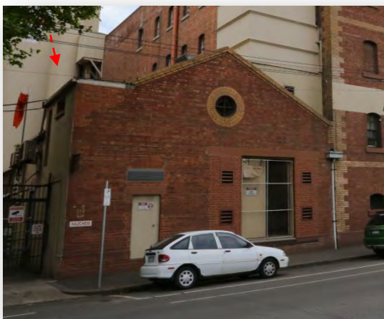
Figure 25 Laurens St, Building 7 2013
