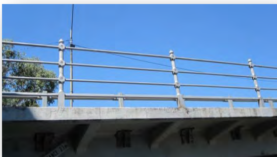
Figure 60 cast and wrought iron balustrade
