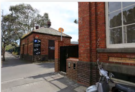
Figure 145 View to north (Google), to caretaker's house (left) now a substation, and regulating house (right), part 98-116 Macaulay Rd
