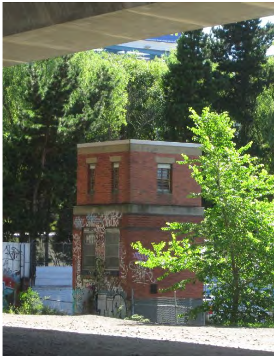
Figure 196 Pump house 2, west end of Sutton Street
