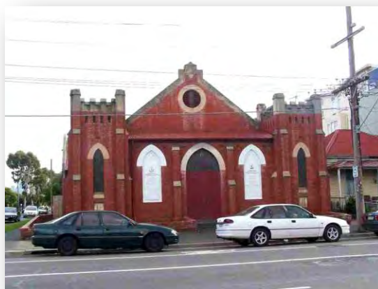
Figure 168 Congregational Church, Burnley Street, RICHMOND, 1920
