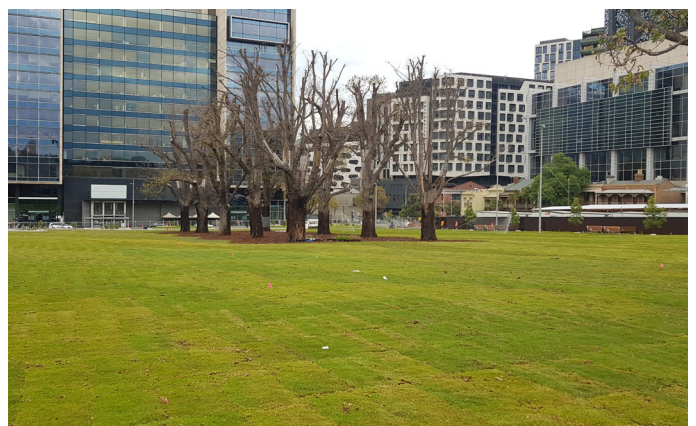
Laying of turf to the central lawn is now complete and will require 13 weeks to fully establish
