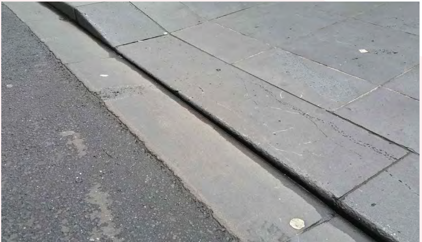
Figure 41: A review of technical notes could address tripping hazards and barriers to wheelchair accessibility across the city, such as this bull-nose ledge.
