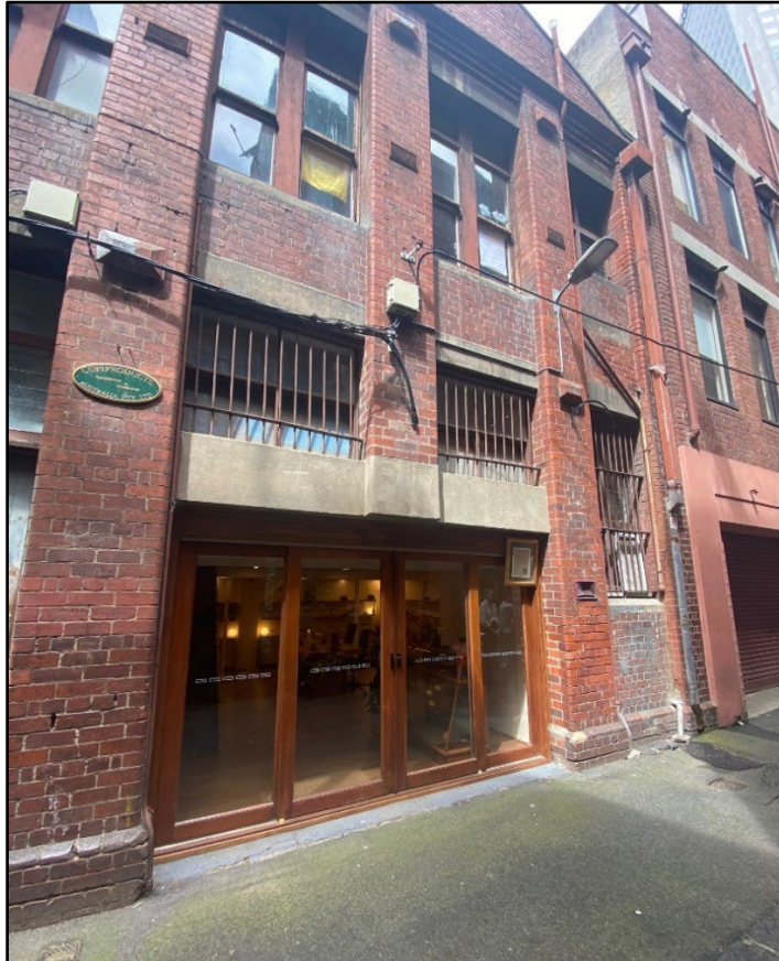
Figure 2: Subject Site from Rankins Lane
