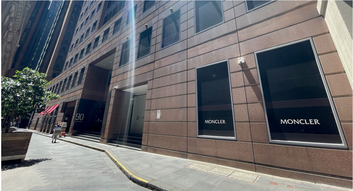
Figure 19 - View of the site from Alfred Place. Captured on 9 December 2022
