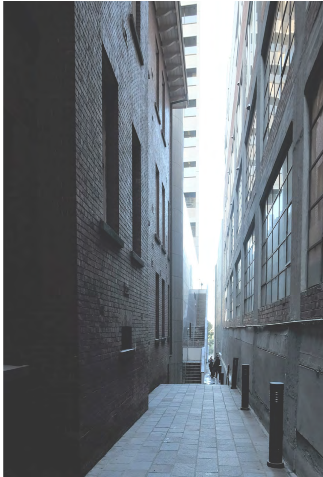
Existing Condition Western Laneway
