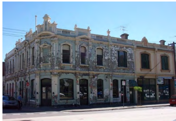
Figure 24 Prince Patrick Hotel, Victoria Parade, Collingwood (HO138 – City of Yarra) Source: Victorian Heritage Database
