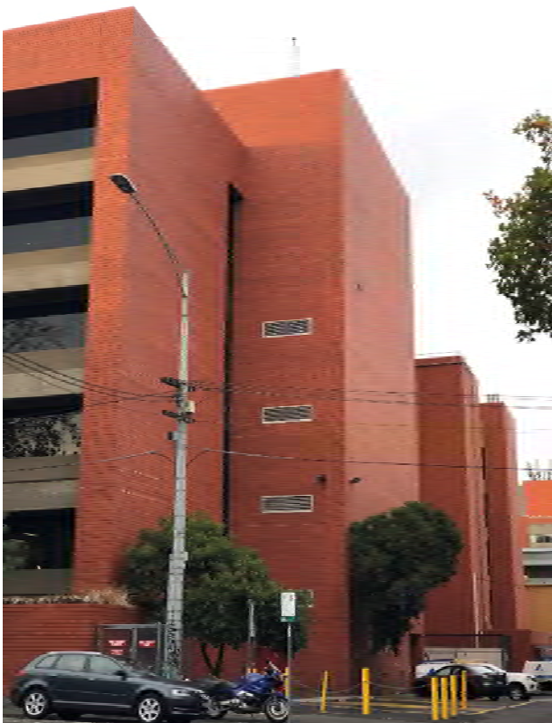
Figure 10 Building 56, west elevation to Little Cardigan Street; the west elevation of Building 57 is in the distance Source: Lovell Chen
