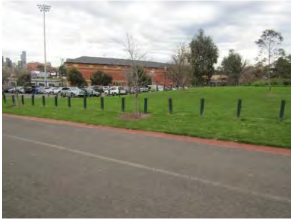
Figure 22. View to the rear of the Jack Dyer Stand approaching from Yarra Park (northeast). (Source: Context-GML 2021 )
