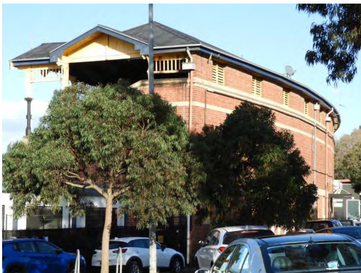
Figure 14. East and the curved north elevation of the Jack Dyer Stand. (Source: Context_GML 2021 )
