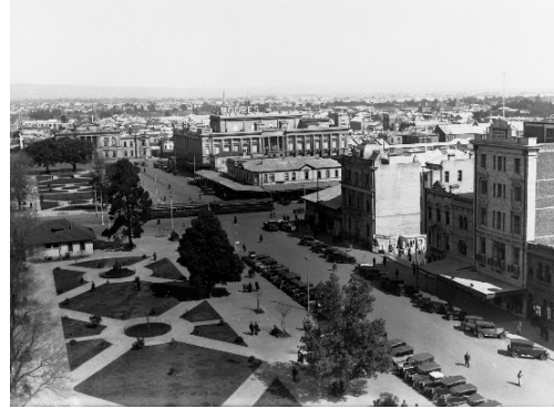
Figure 36 Undated image of Victoria Square/Tarntanyangga, Adelaide Source: http://adelaide.sa.gov.au/places/victoria-square-tarntanyangga
