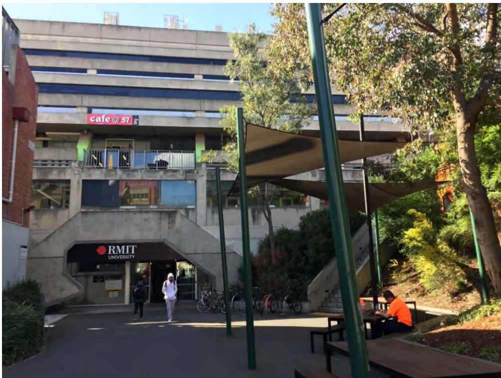
Figure 14 South façade of Building 57, as seen from O'Grady Place, with concrete tiered levels and concrete entrance ramp Source: Lovell Chen
