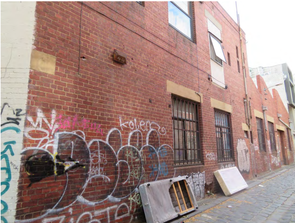
Figure 17 144-146 Queensberry Street, Carlton viewed from Queensberry Lane
