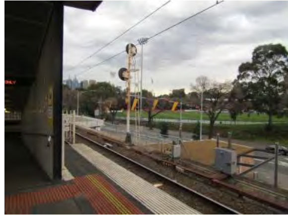
Figure 23. View towards Punt Road Oval from Richmond Railway Station. (Source: Context-GML 2021 )
