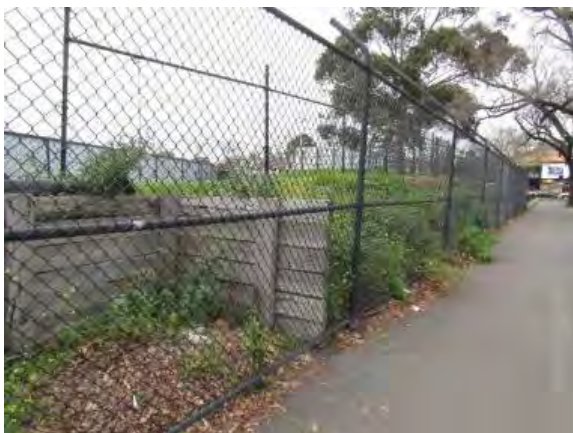
Figure 24. Cyclone fencing, mounding along the Brunton Avenue boundary. (Source: Context-GML 2021 )
