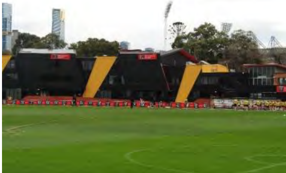
Figure 16. 2011 David Mandie Building (south elevation) facing the ground. (Source: Context-GML 2021 )
