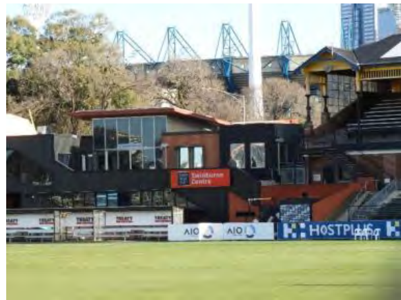
Figure 21. Administration building, with JD Langdon Boardroom. (Source: Context GML 2021 )
