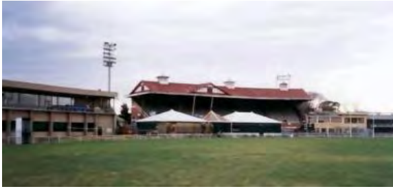
Figure 6. South Melbourne Cricket and Football Club Grandstand, Lakeside Oval, South Melbourne, constructed in 1926 to replace an earlier stand destroyed by fire (National Trust Property No. B6652). (Source: VHD)
