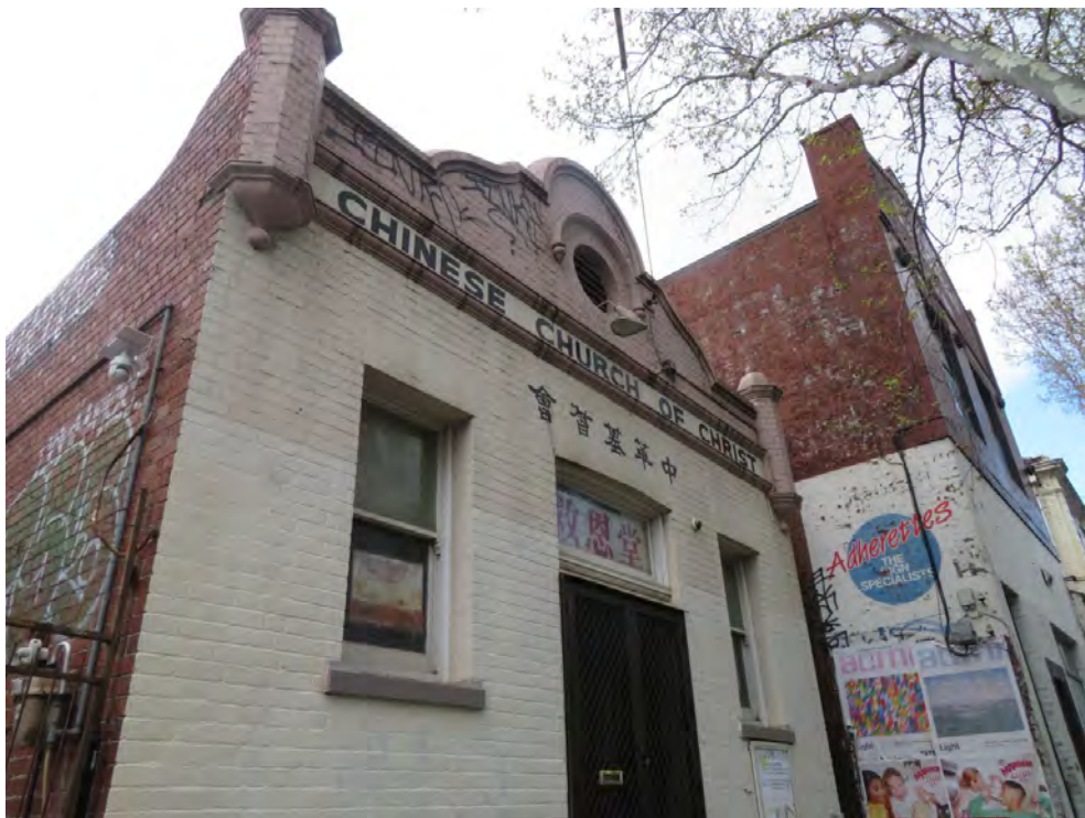
Figure 2 Detail of the principal facade, note the overpainted brickwork and distinctive parapet and pediment Source: Lovell Chen, 2022
