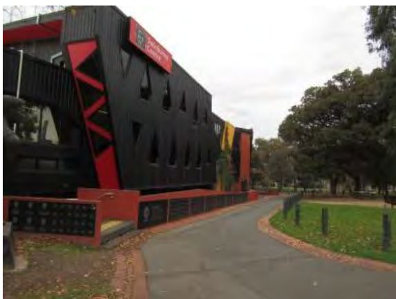
Figure 18. Northern end of the David Mandie Building, with Jack Dyer Foundation Walkway of Honour. (Source: Context-GML 2021 )
