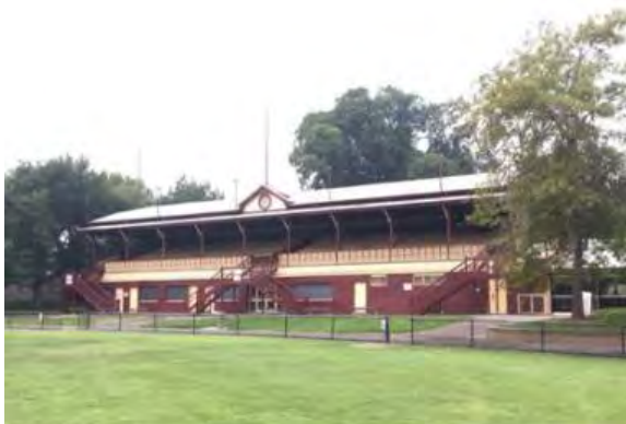
Figure 4. The 1888 Brunswick Street Oval Grandstand, Edinburgh Gardens (HO215, City of Yarra and VHR H0751). (Source: VHD)
