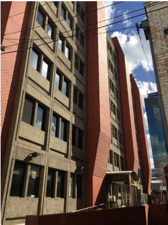
Figure 6 Detail of rear or north elevation of Building 51, with massive brick pilasters or shafts Source: Lovell Chen
