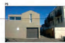
three-storey building to Nicholls lane
