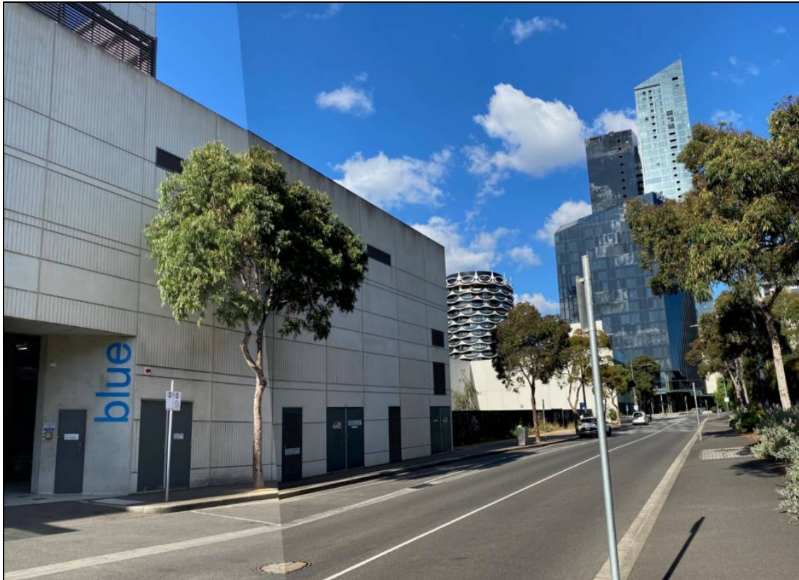
Figure 4: View of the Site along Pearl River Road looking south
