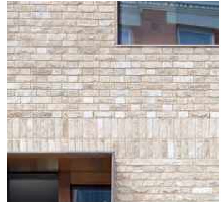
BW01 LIGHT COLOURED BRICKWORK TO PODIUM
