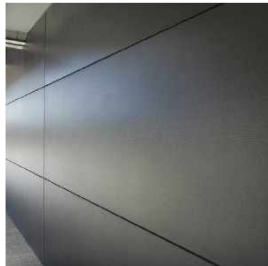
ME07 - WALL CLADDING: GROUND FLOOR ENTRANCE PORTALS
