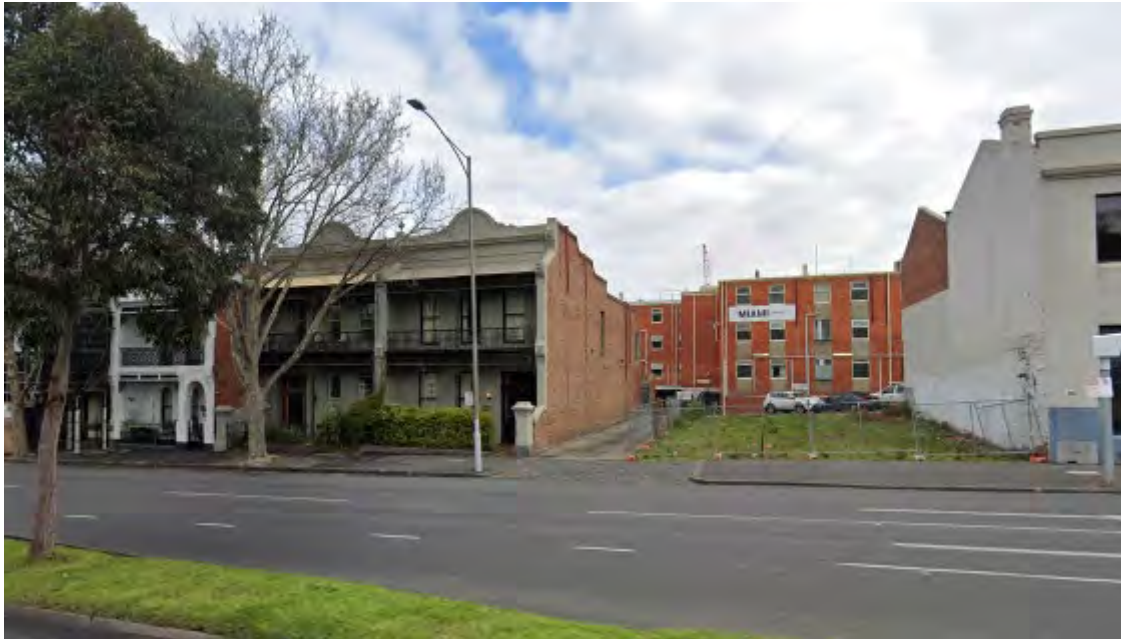
Figure 3: 599-609 King Street, West Melbourne
