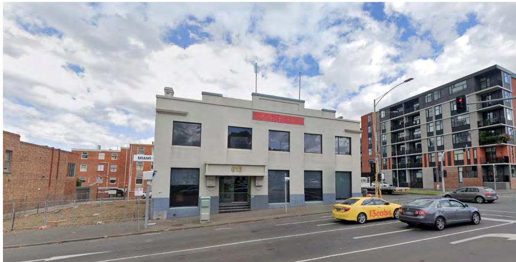
Figure 5: 613 King Street, West Melbourne
