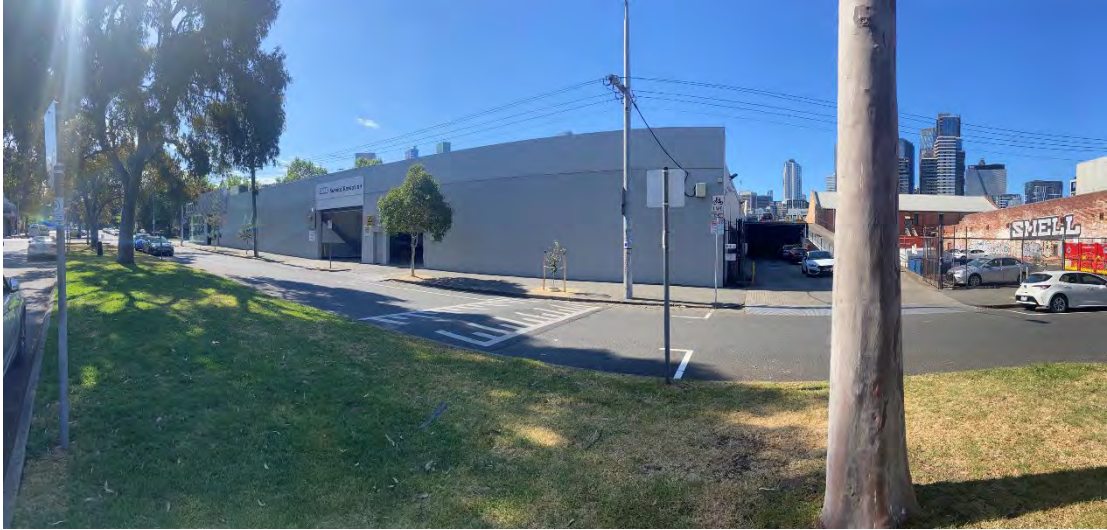
Figure 3 - Roden Street frontage (Council Officers)
