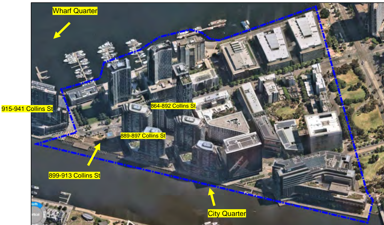
Figure 1 – aerial photograph (dated 1 January 2023) with annotations added by City of Melbourne officers identifying surrounding buildings and the City Quarter and the Wharf Quarter precincts
