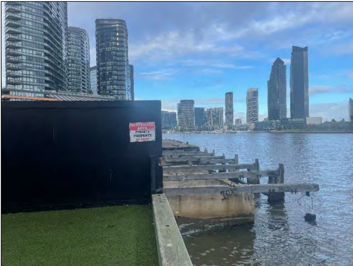
Figure 5 – view to the Australia Wharf facing east (Source: City of Melbourne)
