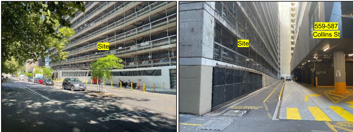
Figures 2 and 3 – view to the Site from Flinders Lane (left) and the view between the Site and 559-587 Collins Street (Source: City of Melbourne, dated 12 February 2024)
