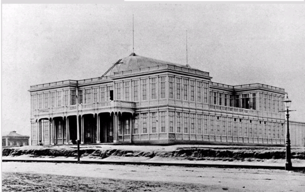
Melbourne's first Exhibition Building on the corner of Little Lonsdale and William Street, 1854
