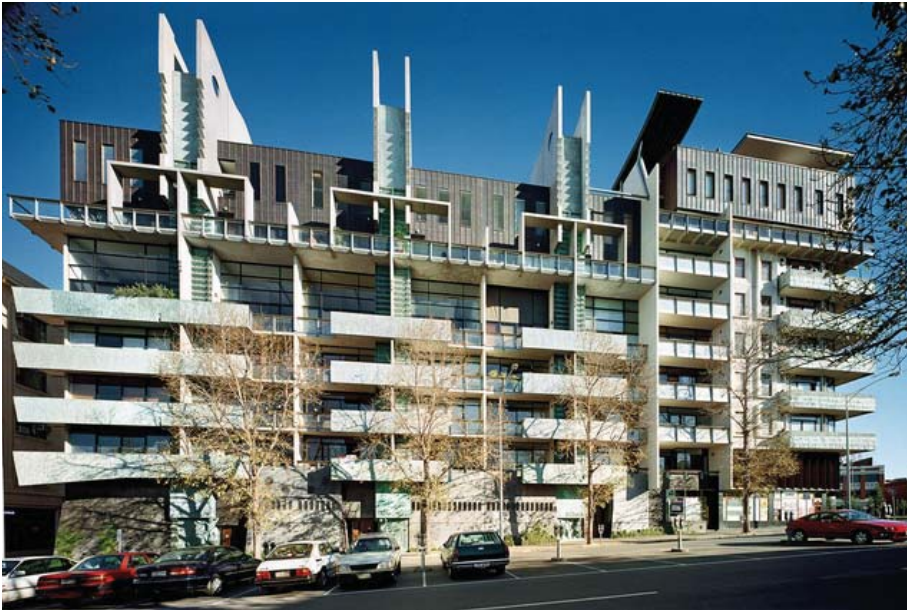
Figure 24. Melbourne Terrace Apartments. [John Gollings, as found at architectureau.com]
