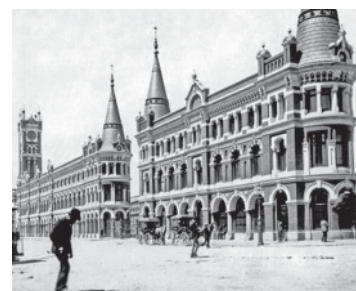
Figure 27. Former Melbourne Fish Market.
