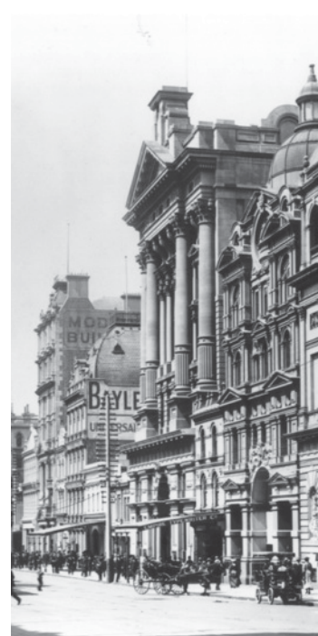
Figure 22. Varied building sizes and styles in Collins Street ca 1900. [N. Caire, National Library of Australia]
