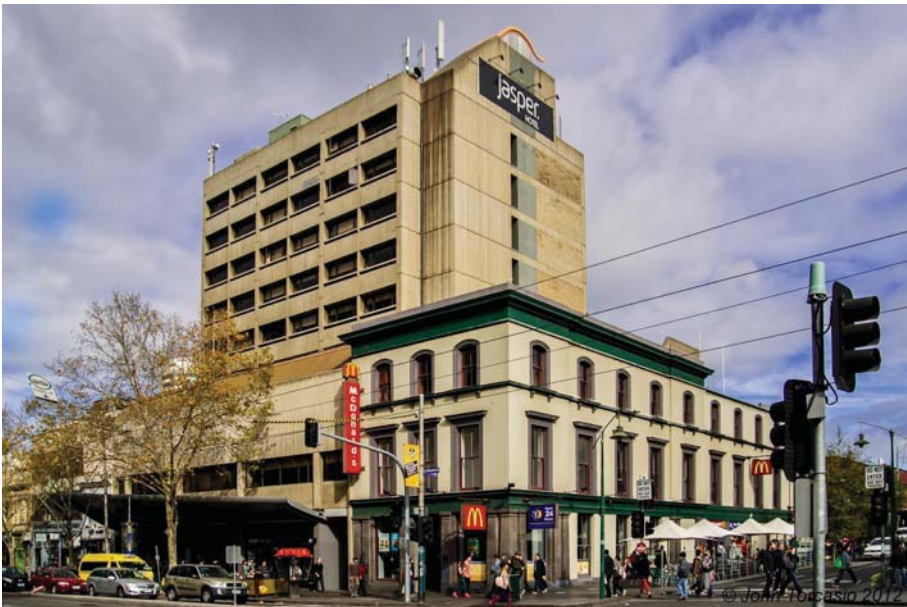
Figure 25. Low-rise retail strip on the west side of Elizabeth Street, including the Jasper Hotel. [John Torcasio, Panoramio.com]
