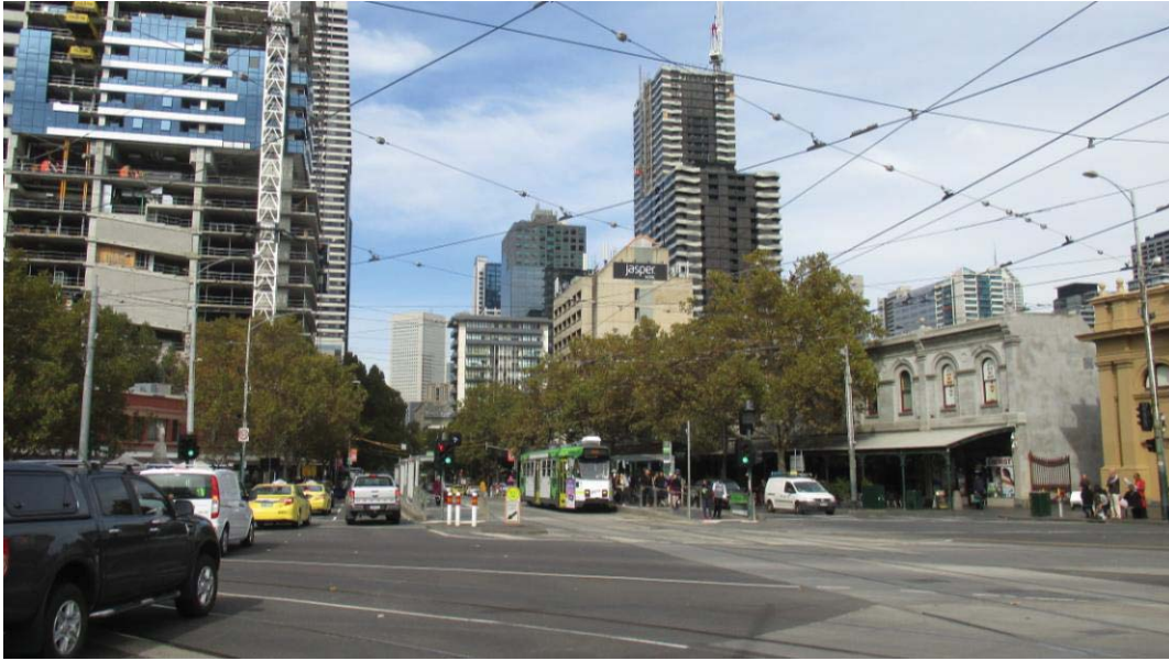
Figure 8 View looking south down Elizabeth Street
