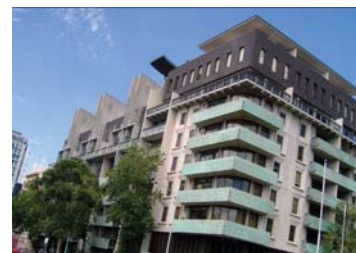
Figure 65. Melbourne Terrace, corner Franklin and Queen Streets
