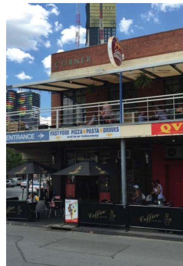
Figure 16. Existing balcony verandah on the Mercat Cross Hotel.
