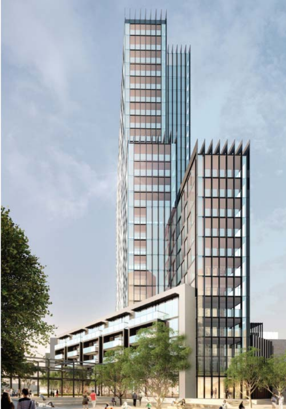
Image 4. View from the northeastern corner of Bourke Dock looking west.
