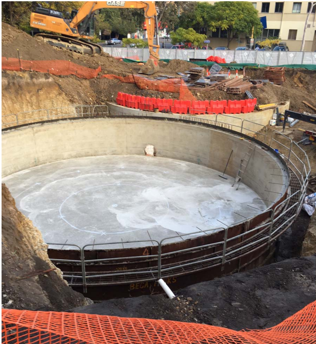
Lincoln Square Storm Water Harvesting and Flood Mitigation Tank
