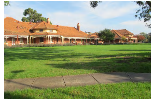
Other development within the Village, including within Stage 1 of the redevelopment (top) and heritage protected buildings on Cade Way (bottom)
