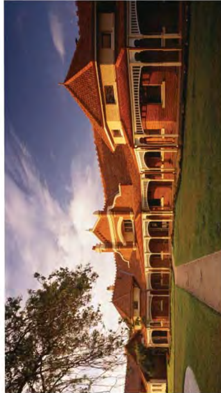
Heritage Precinct buildings adjacent to Subject Site
