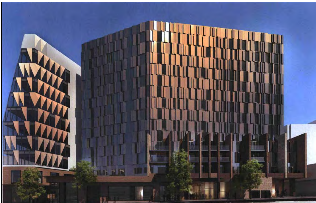
Proposed student accommodation east view – Source: Application documentation
