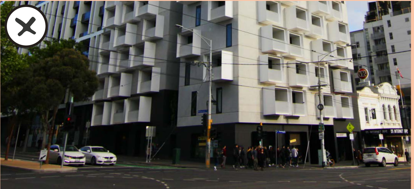
Facade elements which rely on public realm projections as the primary design feature.
