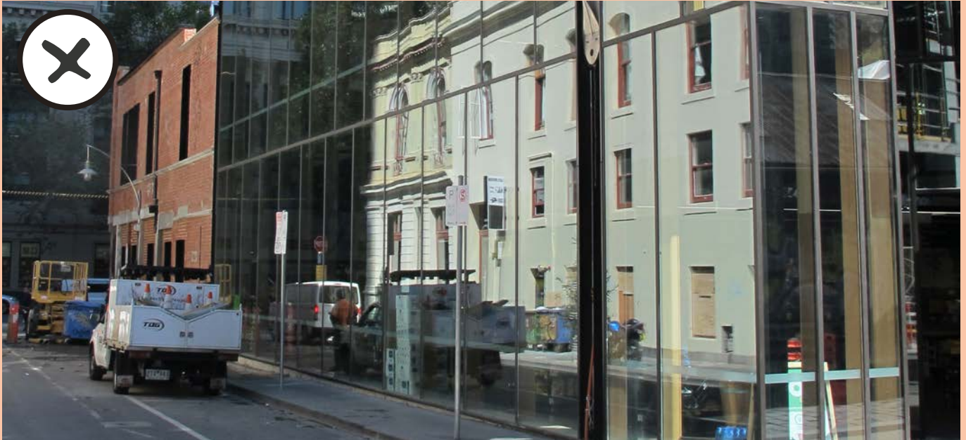
The use of tinted, opaque or high reflectivity glass which obscures views between the public realm and building interior within the lower levels of a building.
