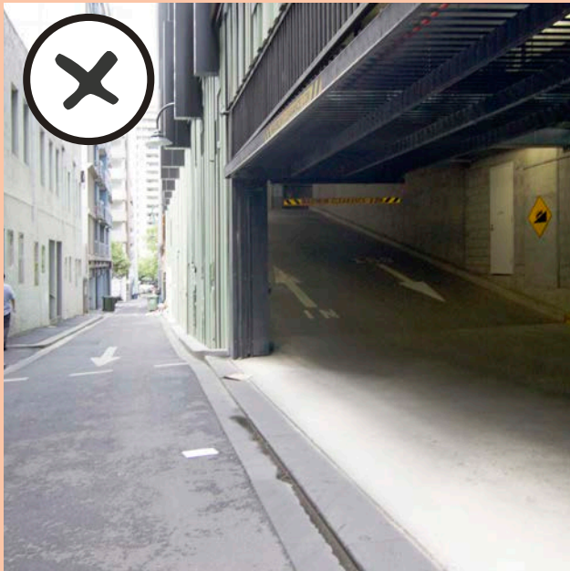
Ramped parking structures which preclude adaptation for other uses.
