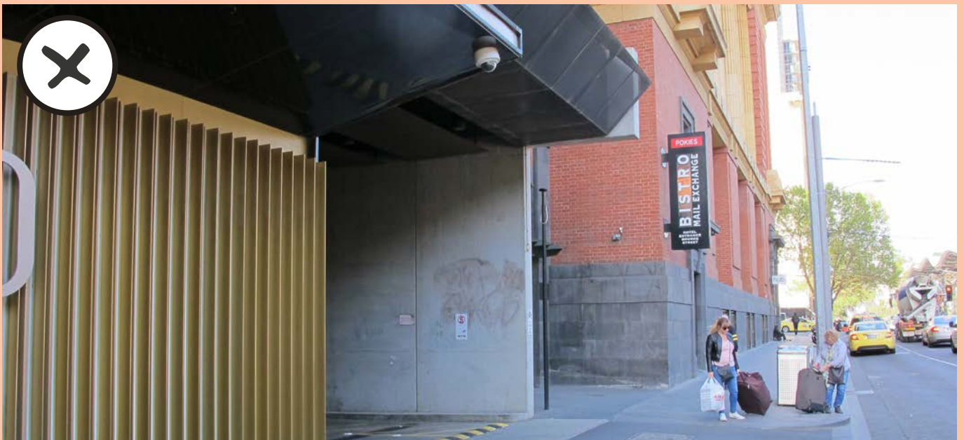
Small, narrow publicly accessible spaces, alcoves and recesses that lack a clear public purpose.
