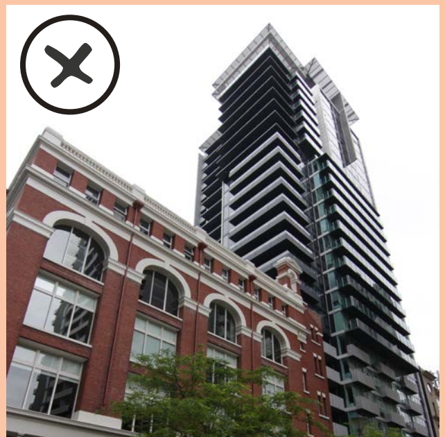
The use of flat facades with reliance on surface or decorative effects where a setback is required to achieve a transitional in height and mass to an adjacent heritage place or precinct.
