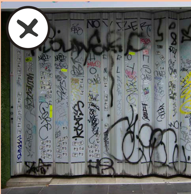
Opaque or translucent security installations which obscure views into tenancies at night.
