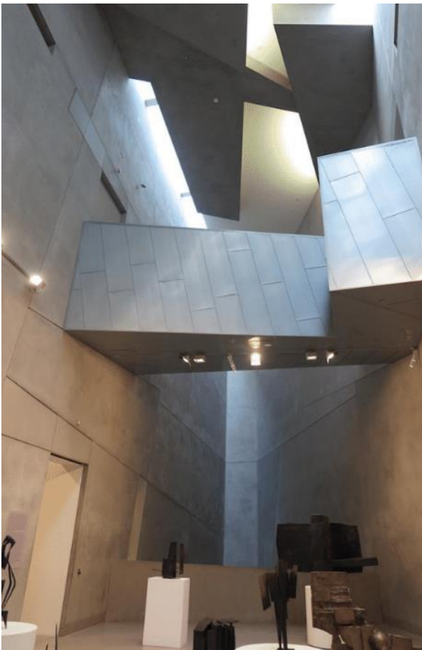
2018, Ian Potter Centre: NGV Australia sculpture gallery with zinc panelling and plastered walls.
