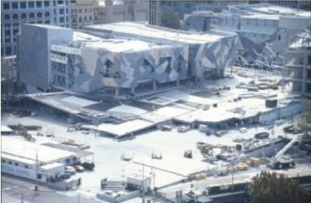
Decking under construction. Source: LAB Architecture Studio
