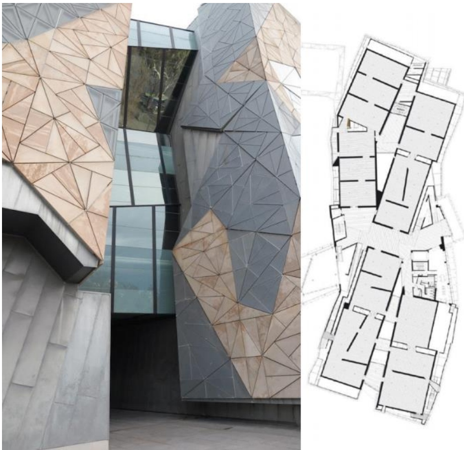
2018, Southern side of Ian Potter Centre: NGV Australia showing glazed spaces between filaments, and plan of NGV.
