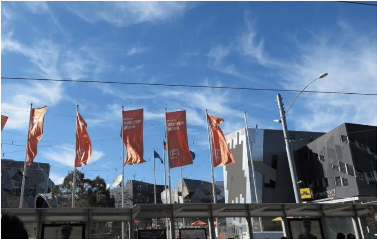
2018, Swanston Street elevation (buildings left to right: Alfred Deakin Building, Crossbar, Yarra Transport, connected by catenary lighting system).
