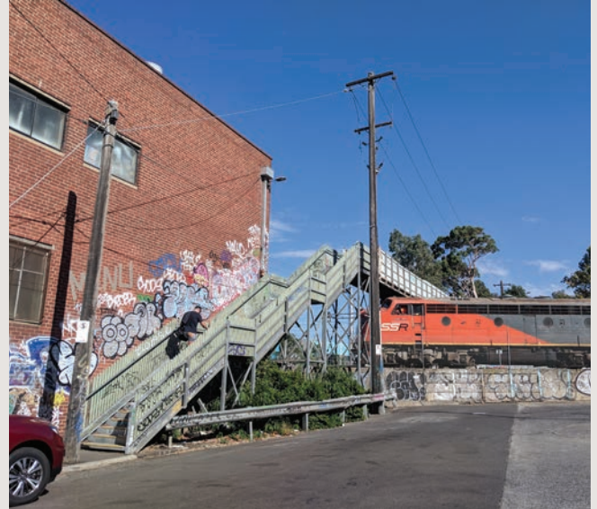
Figure 1.40: Photo of existing footbridge over the Kensington Railway, subject to HO638
