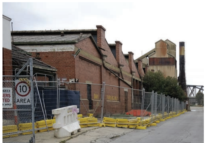
Figure 1.17: Example of a sawtooth warehouse, located at 1-39 Hobsons Road. The site was originally used for meat processing and noxious trade. (Number 3 on map)
