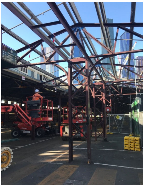
Image: Roof replacement works in L Shed
