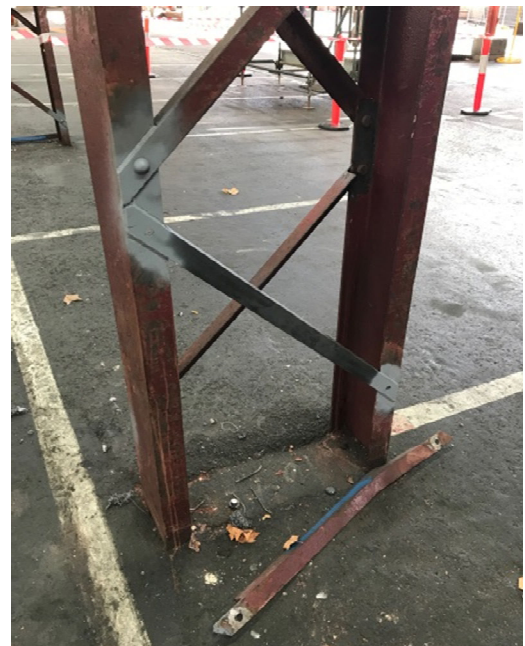
Image: Structural repairs
