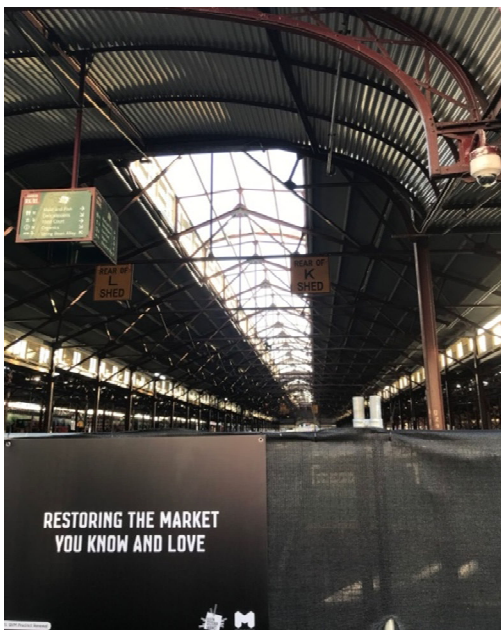
Image: Roof replacement works in rear of K and L sheds
